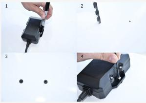
2. If power cable needs to breach asset housing, utilize the provided grommet and butt connectors.
